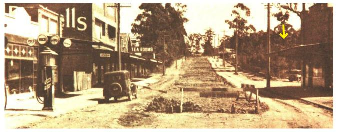
Figure 2.8 'Preparing Pennant Hills Road for concreting, 1929. Fisher Ave on right'. View west along Pennant Hills Road with subject site indicated by
